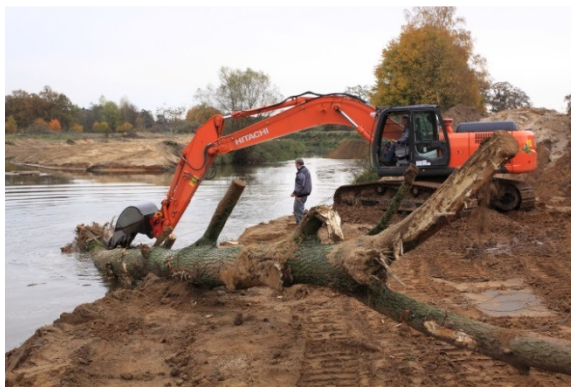
Totholzeinbau Incorporation of dead wood
